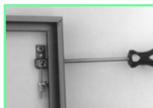
**Step 3:** Lock the hanger by tightening the locking screws with a screwdriver. It's that easy!
